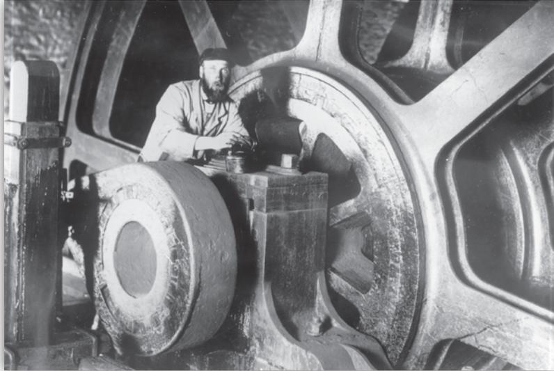
In the 1890s, the machinery was operated by the winding engine driver Jimmy Hoil. The triangular crank you can see in the photograph attached to the eastern end of the drum's axle meant that as the drums turned, the water was supplied to the locomotive and stationary pumping engine. Photograph courtesy of Mike Jones.
